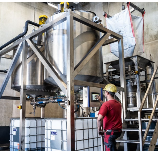
The premix is prepared for dispersing in large steel tanks.
